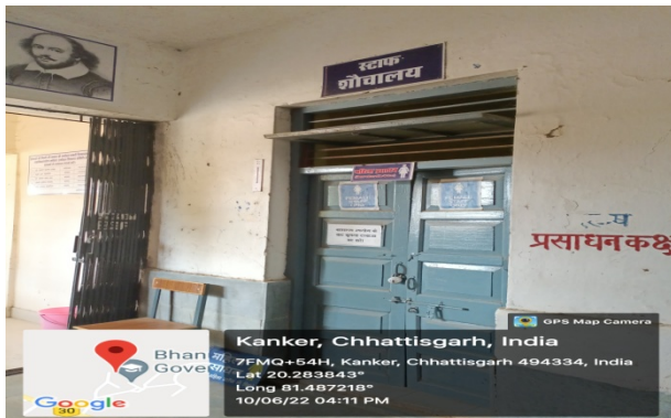
Wash Room for Ladies Staff
